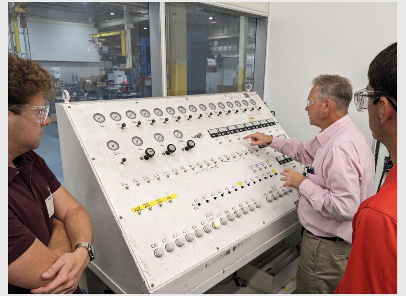
Existing simulator: Large analog switchboard
