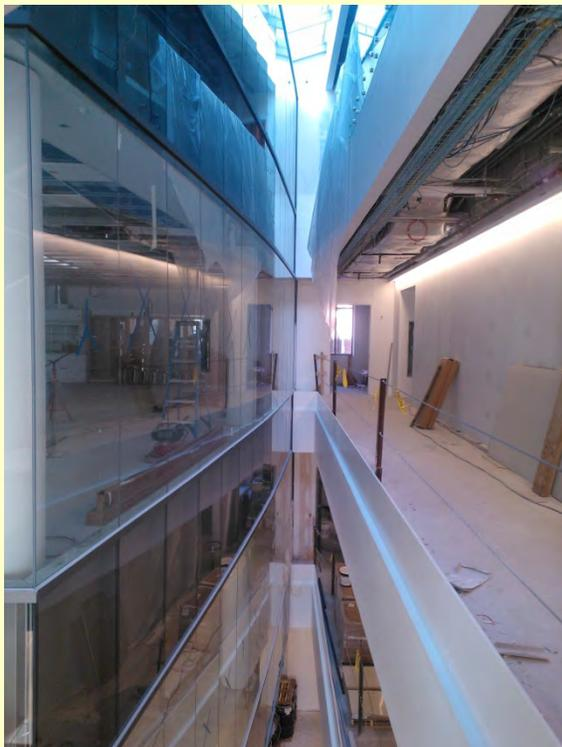
The picture at left shows off two of the dominant features of STEM Hall. To allow natural light throughout the building, there will be open areas from the basement up to the third floor, between the hallways and the main labs located in the center of the building. To allow this light into more of the building, there are many interior windows. This also allows for “science in sight” – as visitors go through the building, from the hallways they will have full view of what’s happening in the labs.
