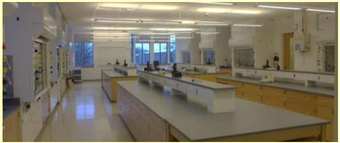
Some of the most significant upgrades in the new Organic Lab are the 12, five-foot ventilation hoods located around the perimeter of the lab. They are large enough to be used by two students, so that this lab can hold up to 20 students with each being able to work in a hood. The benches are arranged so that individual lab drawers are situated near to the hoods, and students will work around the perimeter benches. The interior benches are then available for instruments, balances, etc.
