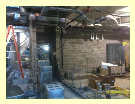
This picture shows how the mechanical systems are underway, with piping for utilities being installed. The cement block wall shown will house the elevator shaft.
